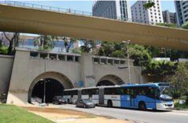
Construction of viaducts, tunnels or other improvements
